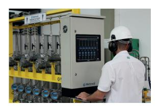
Monitoring of all variables, complete reading of data, injection control alarms, remote calibrations of Control Valves carried out through a dedicated panel, PLC (programmed logic controller), in turn, commands a special needle valve with electric actuator, through previously determined opening and closing, give the exact value to be injected in the corresponding oil line.
